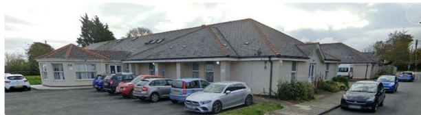
The first of many nursing homes built in the early nineties. The first to have single room with en-suites and hospital level common services and is now the format for all new nursing homes of today.
